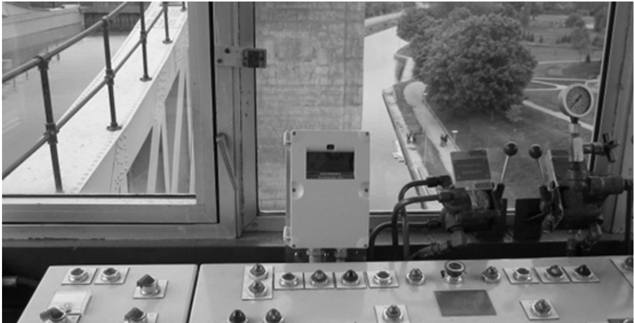
MultiRanger measuring canal levels at Peterborough Lift Lock, Ontario, Canada
